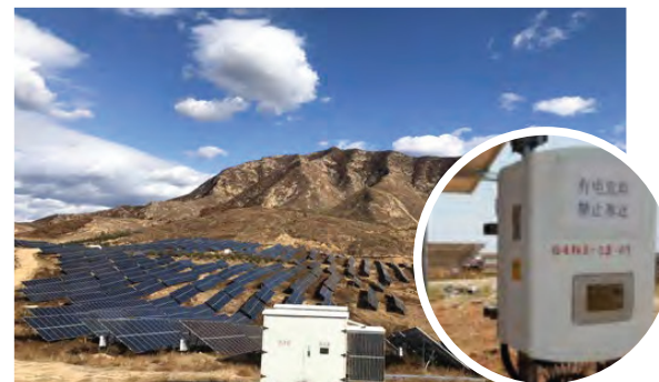
*Liaoning Gaizhou Jiuzhai PV Plant 20MW
