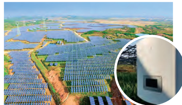
*Zhejiang Hangbu Agricultural-photovoltaic hybrid PV Plant 30MW
