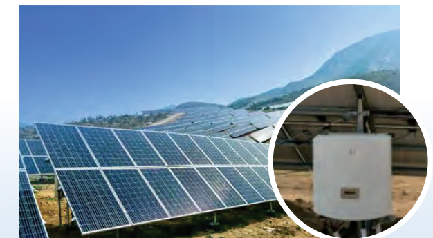
*Liaoning Yingkou Jiuzhai PV Plant 20MW
