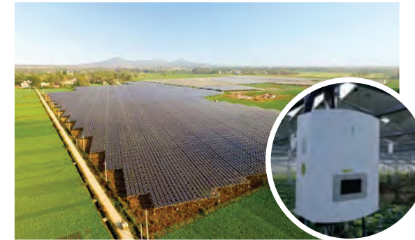
*Hubei Guanyin Agricultural-photovoltaic hybrid PV Plant 20MW
