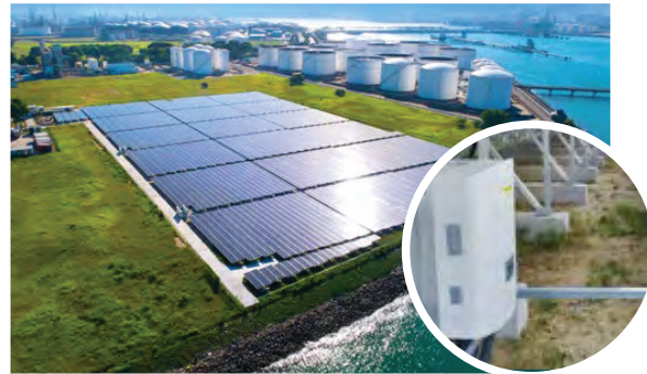
*JTC Solar Farm, Singapore 5MW
