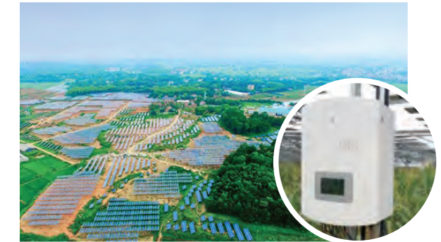
*Quzhou Qinghu Agricultural-photovoltaic hybrid PV Plant 20MW
